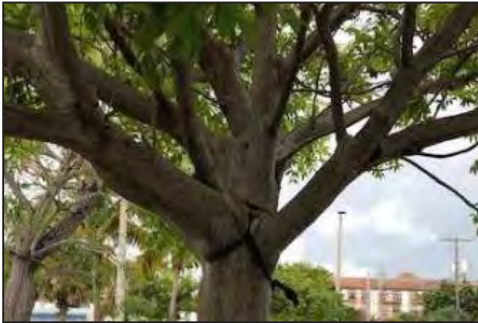
Photo 33. The staking and guying material was not removed or adjusted one year after planting and is now girdling the stem. This is an example of poor maintenance.
